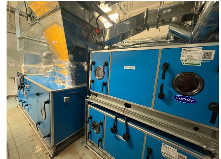
New AHU installed in RAC Lab
